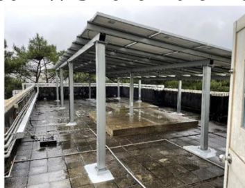
Installation of Solar Panel
